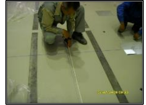
Marking lines for embedded base
