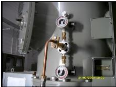
Vacuuming before the gassing works
