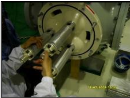
Cleaning internal parts of docking points
