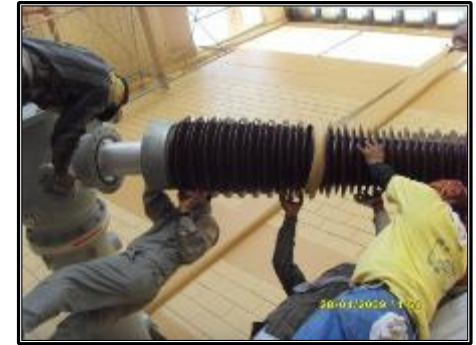
Assembling Gas to Air bushing
