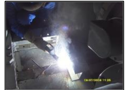
Welding all bays to embedded base
